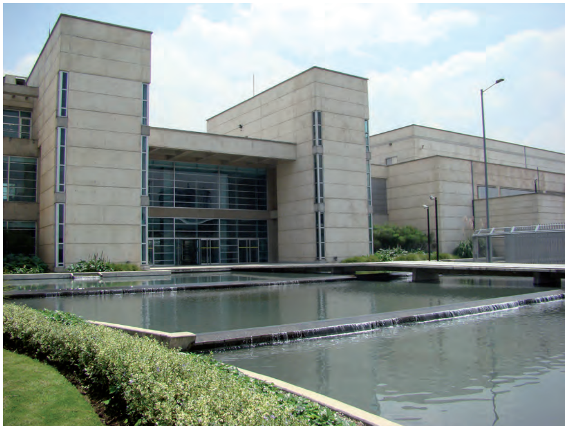
The water pool at the Central de Efectivo collects rainwater, which is used for toilets, garden irrigation, and as a reservoir for the firefighting system.
